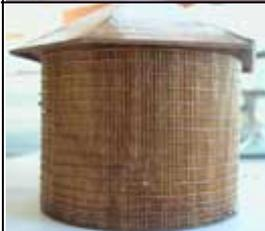
Using electric brass wire, wind it around the tank and twist together the end to tighten narrow the tank wall. Leave more or less 5 twist, cut the excess and turn parallel the wall. The band at bottom should be closer together than the top ones.
